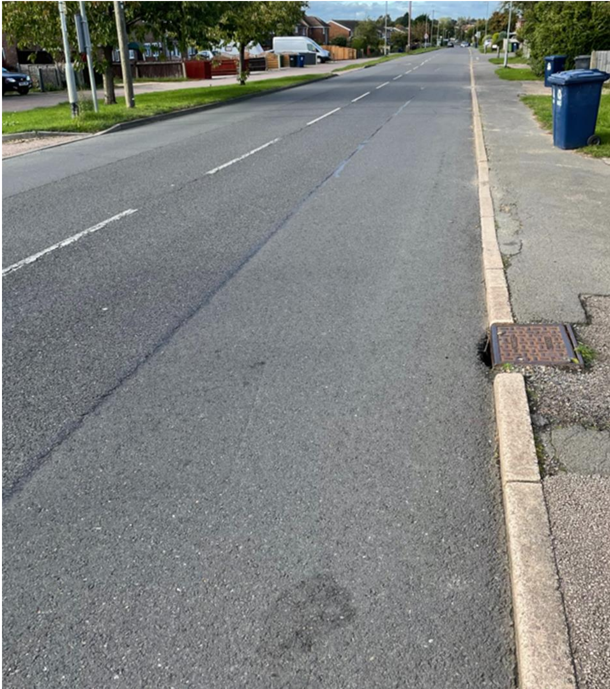
Figure 9: Photo of B1046, NW of railway bridge. 6.8m carriageway, kerbed
