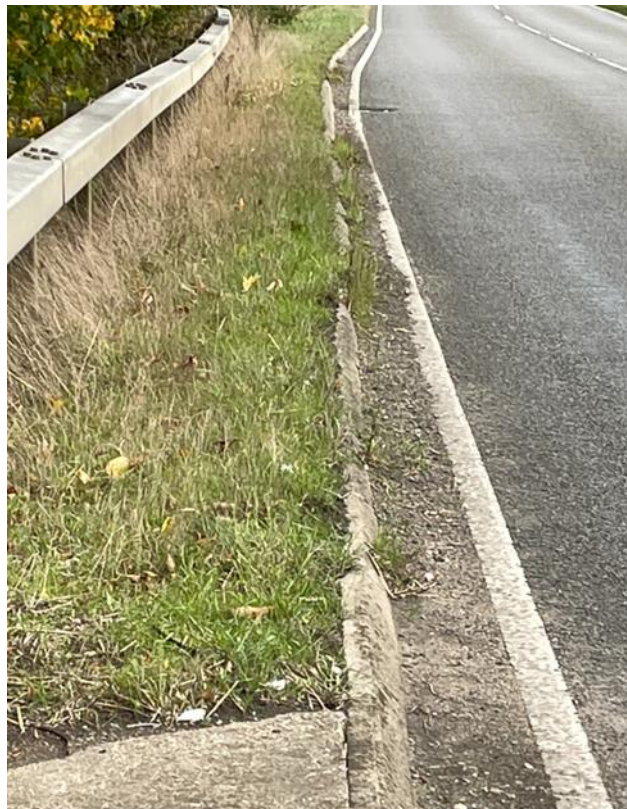
Figure 11: Photo of B1046 at bridge over existing A428
