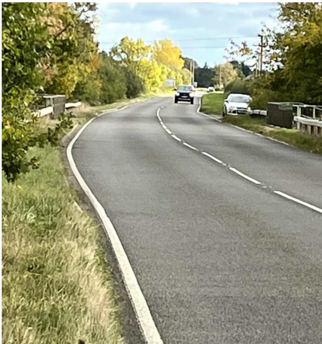
Figure 12: B1046 at bridge over existing A428
