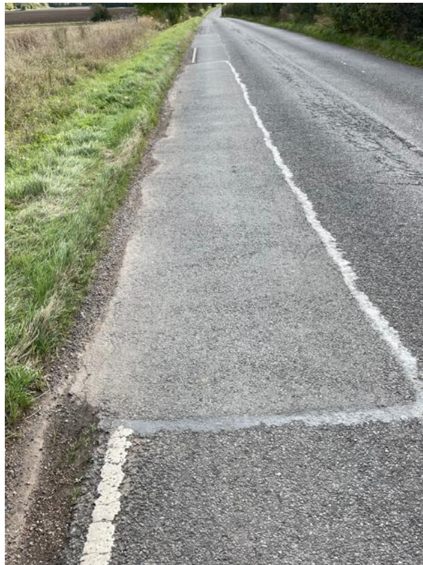
Figure 3: Typical edge repair, Toseland Road
